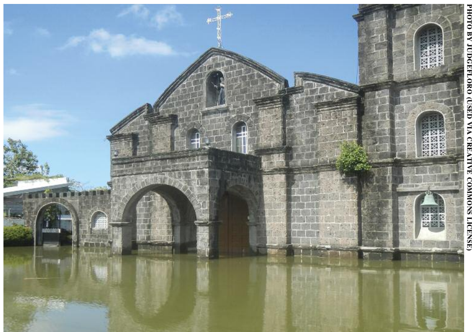
VULNERABLE PLACES: Saint Monica Chapel in Hagonoy, Philippines, just north of Manila, during a flood in October 2020.
