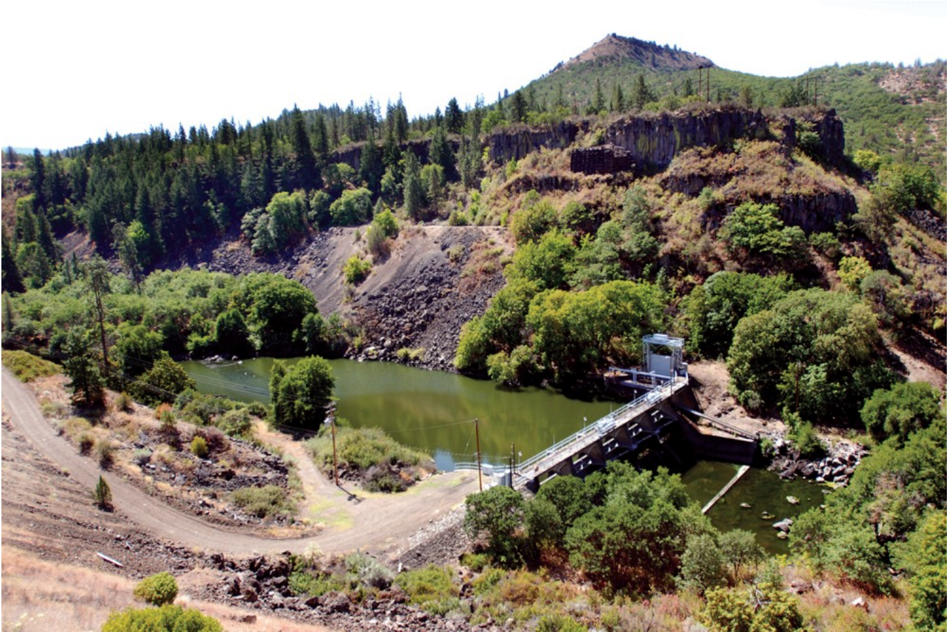
The Copco 2 hydroelectric dam on the Klamath River, outside Hornbrook, California, prior to its removal in July 2023. (AP photo / Jeff Barnard / File)
